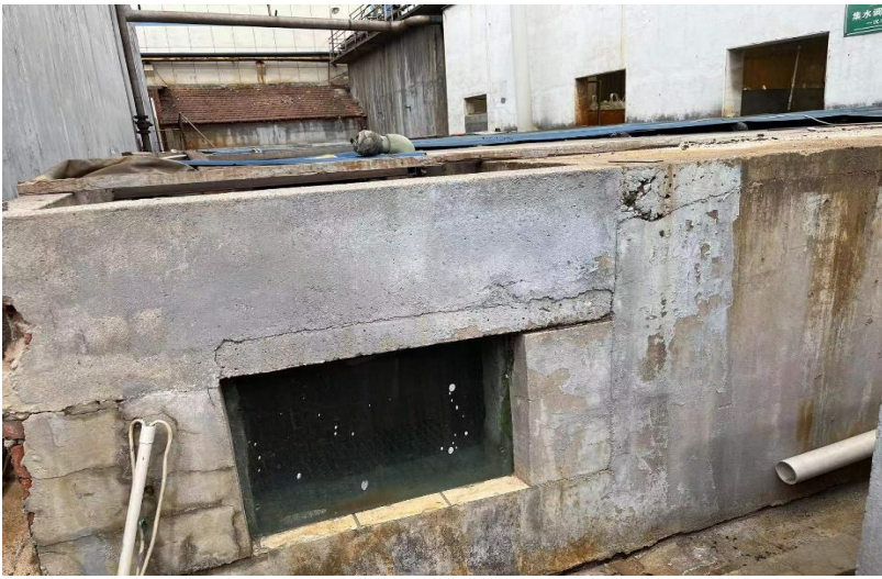
Photo of before treatment area
