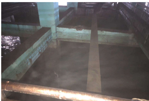
Photo of before treatment area
