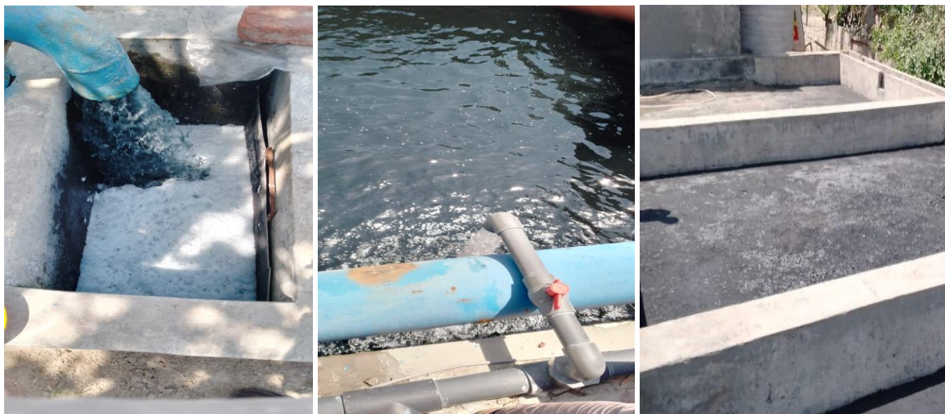
Sampling Point - Untreated Wastewater
