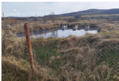
Photo of Sludge Area
