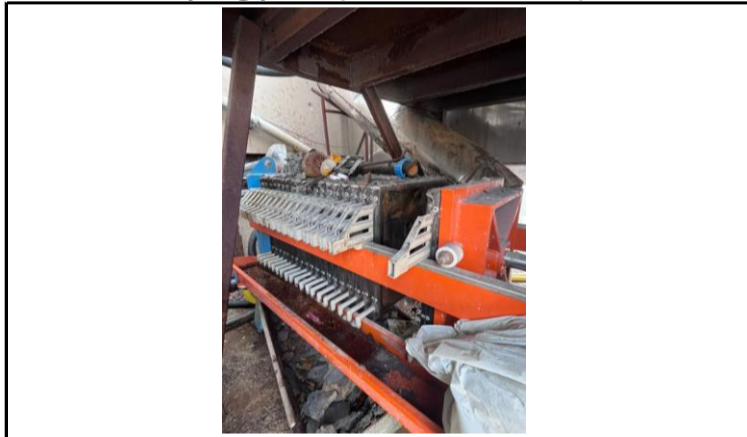
Photo of Sludge Area
