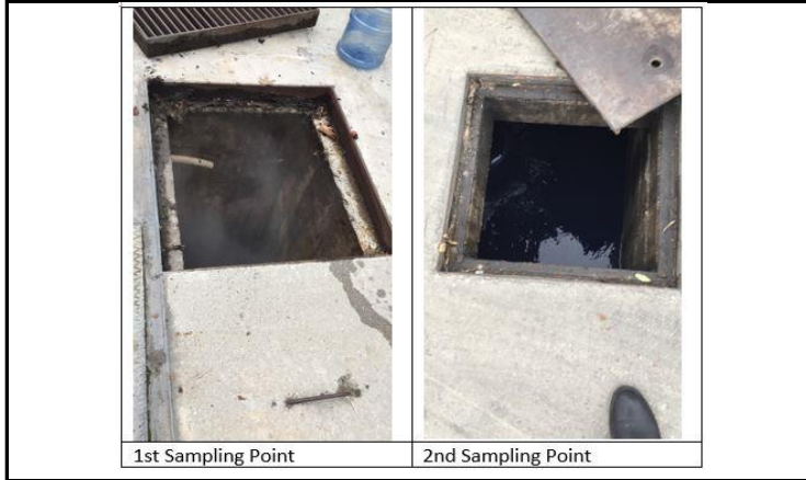
Photo of before treatment area
