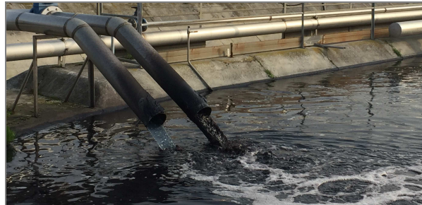
Raw Wastewater (Before Treatment Plant)
