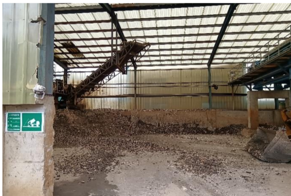
Photo of Sludge Area
