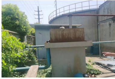
Photo of wastewater after treatment area
