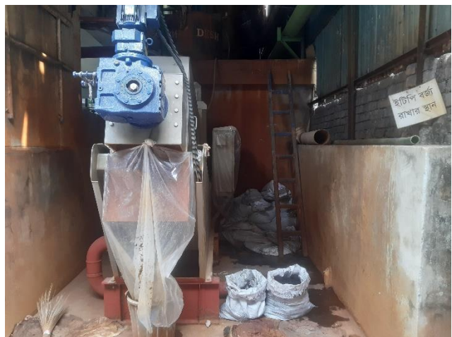
Sludge Bed (GPS location: Latitude 23.919148, Longitude: 90.387781)
