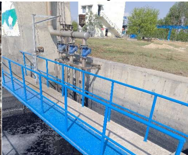
I001) Sampling location surrounding Lat 30.9087, Long 76.130752
