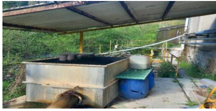
Photo of before treatment area
