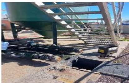
Photo of Sludge Area
