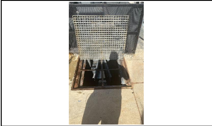
Photo of before treatment area
