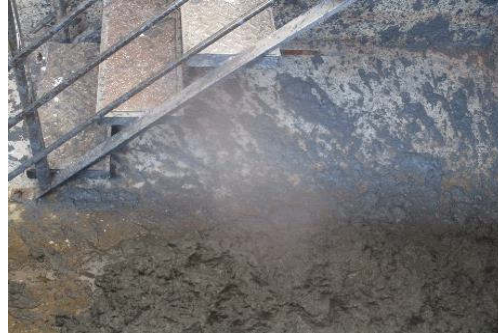
Sampling point surrounding environment 22/09/2024; 16:13
