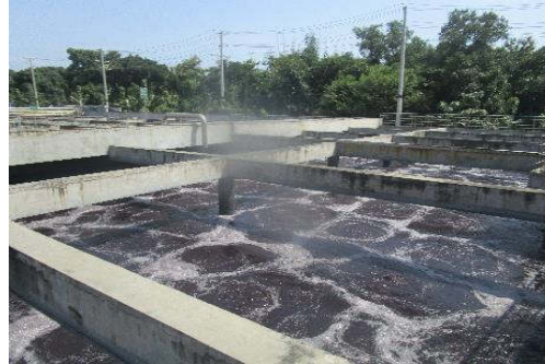
Sampling point surrounding environment 22/09/2024; 16:25
