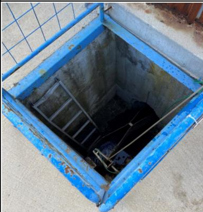
SAMPLING LOCATION, CLOSE-UP VIEW
