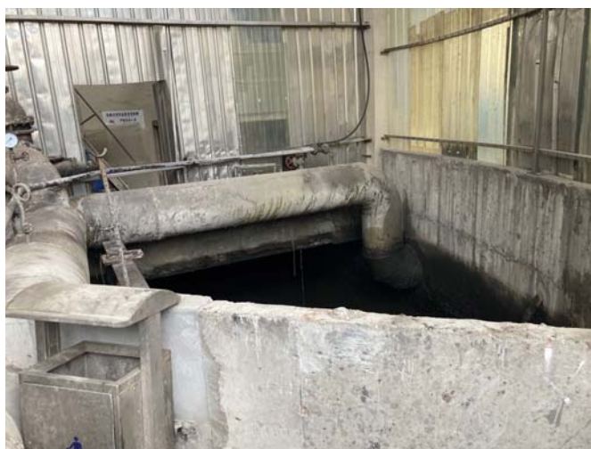
Photo of before Treatment Area
