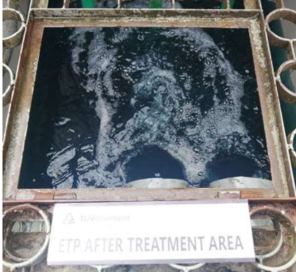
Fig- Foam in Aeration Tank
