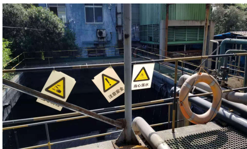
Photo of before treatment area
