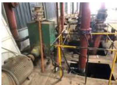
Photo of before treatment area
