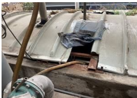
Photo of before treatment area
