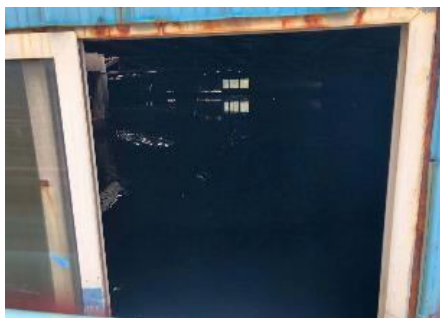
Photo of before treatment area
