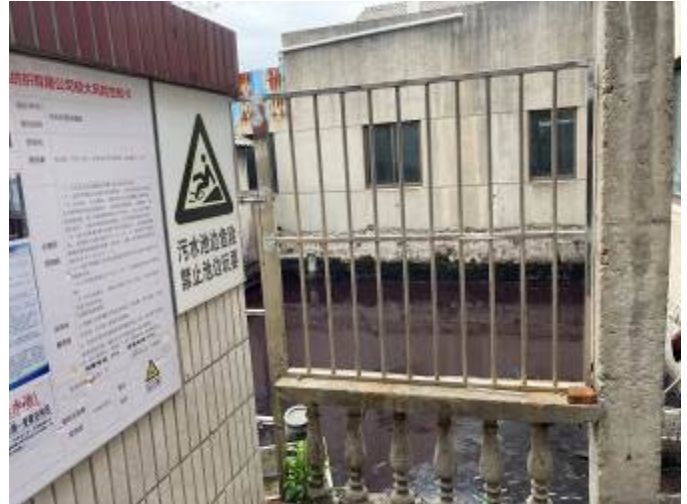
Photo of Before Treatment Area
