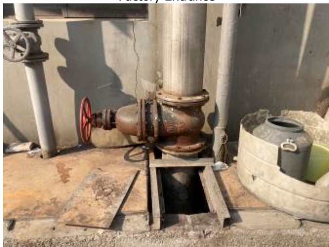
Photo of Before Treatment Area
