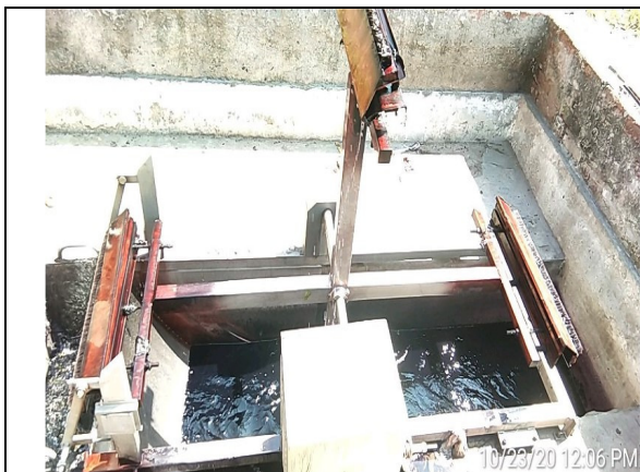
Photo of sampling point (Raw wastewater)
