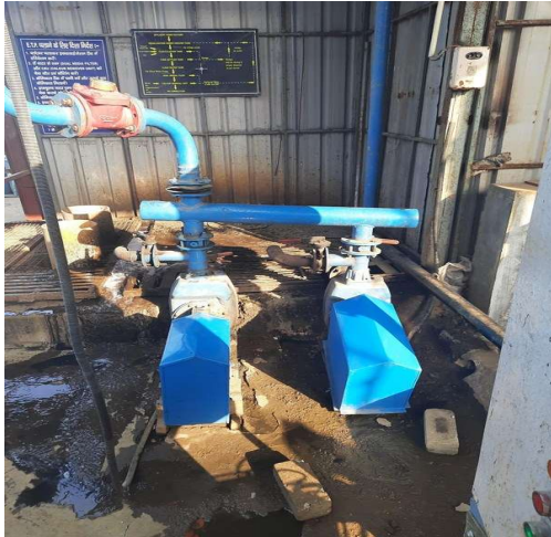
Photo of before treatment area
