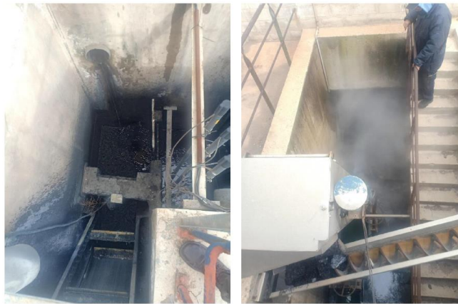
Photo of before treatment area
