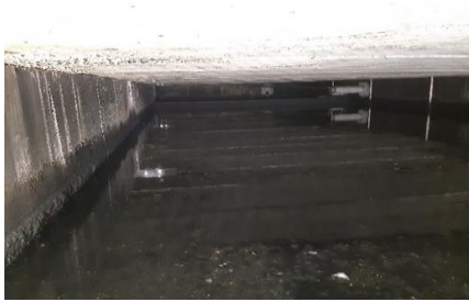
Photo of before treatment area
