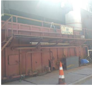
Photo of before treatment area
