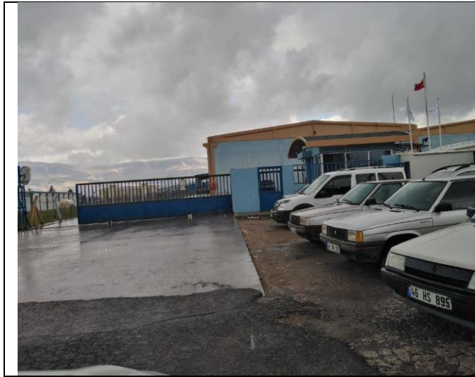
Front of the production unit
