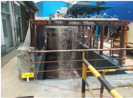
Photo of before treatment area
