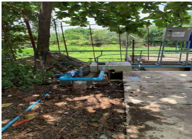
Raw Wastewater Collection Area
