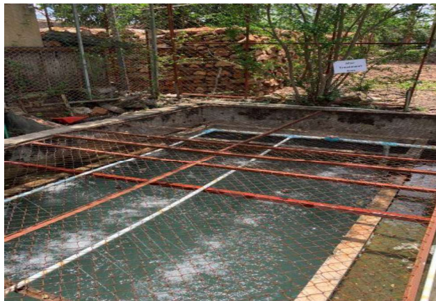
Treated Wastewater Collection Area
