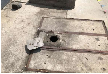
Photo of before treatment area
