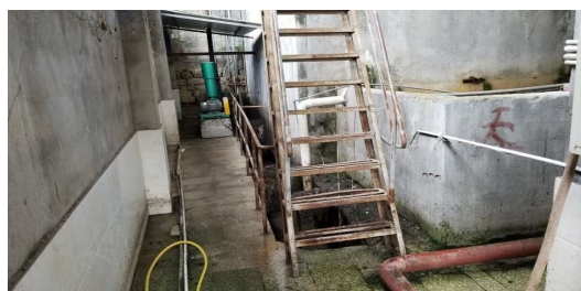
Photo of before treatment area
