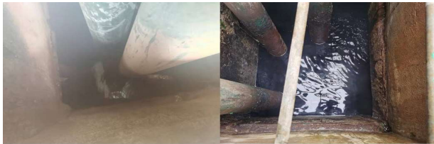
High-Concentration Low-Concentration Photo of sampling point (before treatment)
