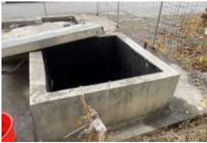
Photo of before treatment area
