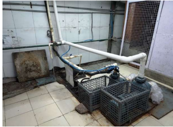
Photo of before treatment area
