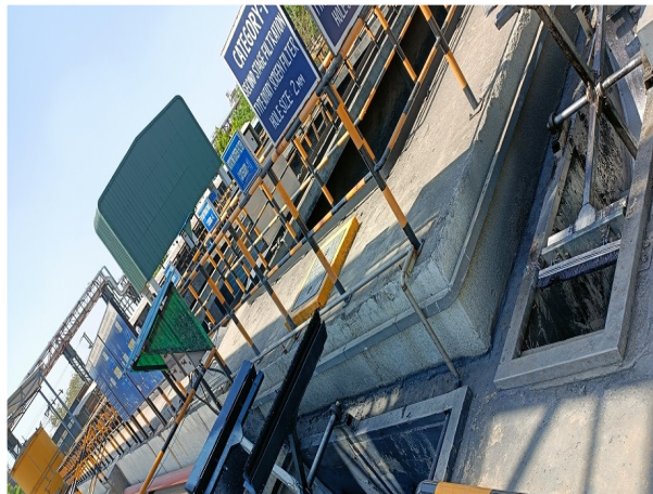
Photo of sampling point Sample -2 (Raw Wastewater-Low TDS (Unit- 2))
