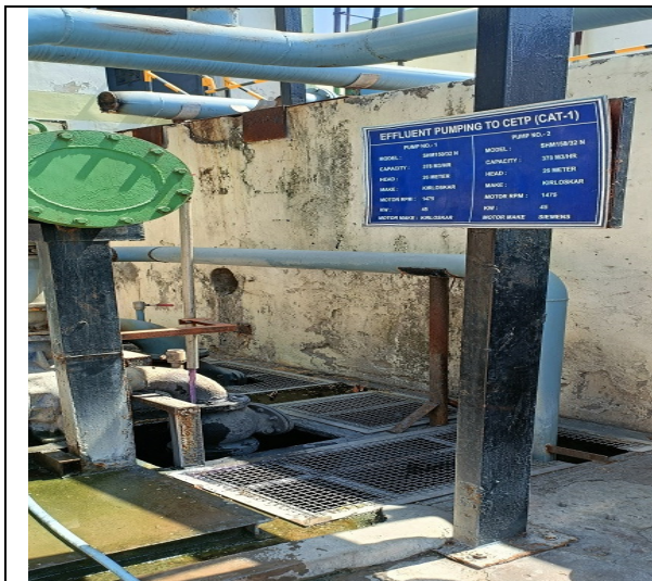
Photo of sampling point Sample -1 (Raw Wastewater-Low TDS (Unit- 1))
