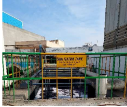
Photo of before treatment area
