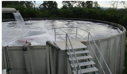
Photo of before treatment area
