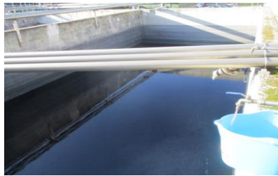
Photo of before treatment area
