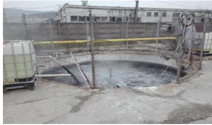
Photo of before treatment area
