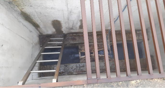
Photo of before treatment area
